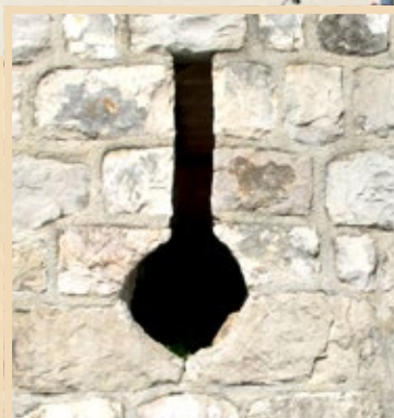
Puškarnica »na ključanicu« u cavtatskim zidinama, 15. st. / Keyhole-style loophole (gun slit) in the walls of Cavtat, 15 th ct.
